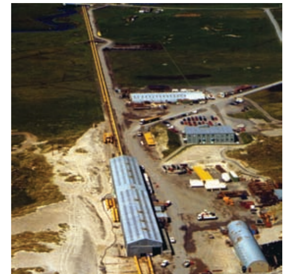
WICK BUNDLE FABRICATION YARD UK
