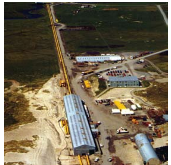
WICK BUNDLE FABRICATION YARD UK
