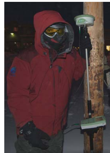
Fig. 2: GPS measurements of the piles
