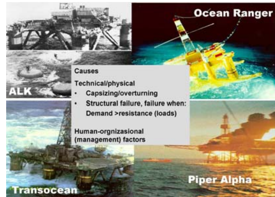
Fig. 40 Offshore accidents. Alexander L. Kielland (ALK): fatigue failure of brace, loss of buoyancy and capsizing. Ocean Ranger: accidental flooding and capsizing. Transocean: explosion. Piper Alpha: fire and explosion
