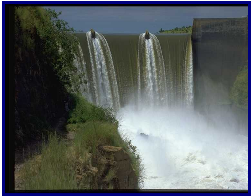
Cambambe Dam, River Kwanza, Angola
