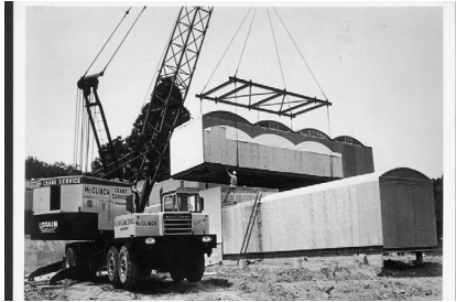
Fig. 1 - View from construction phase
