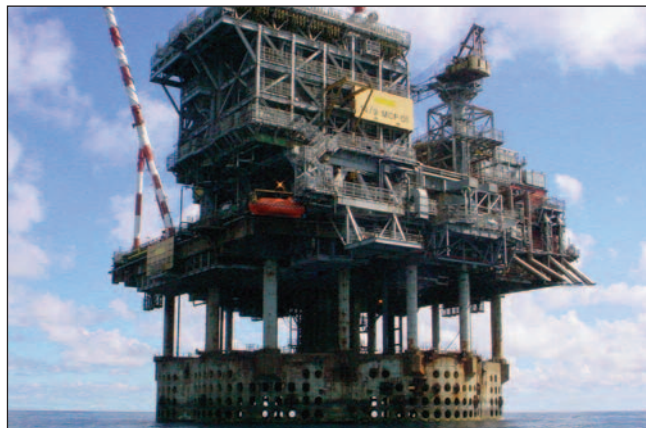
Figure 6.2 MCP-01 Topside facilities
