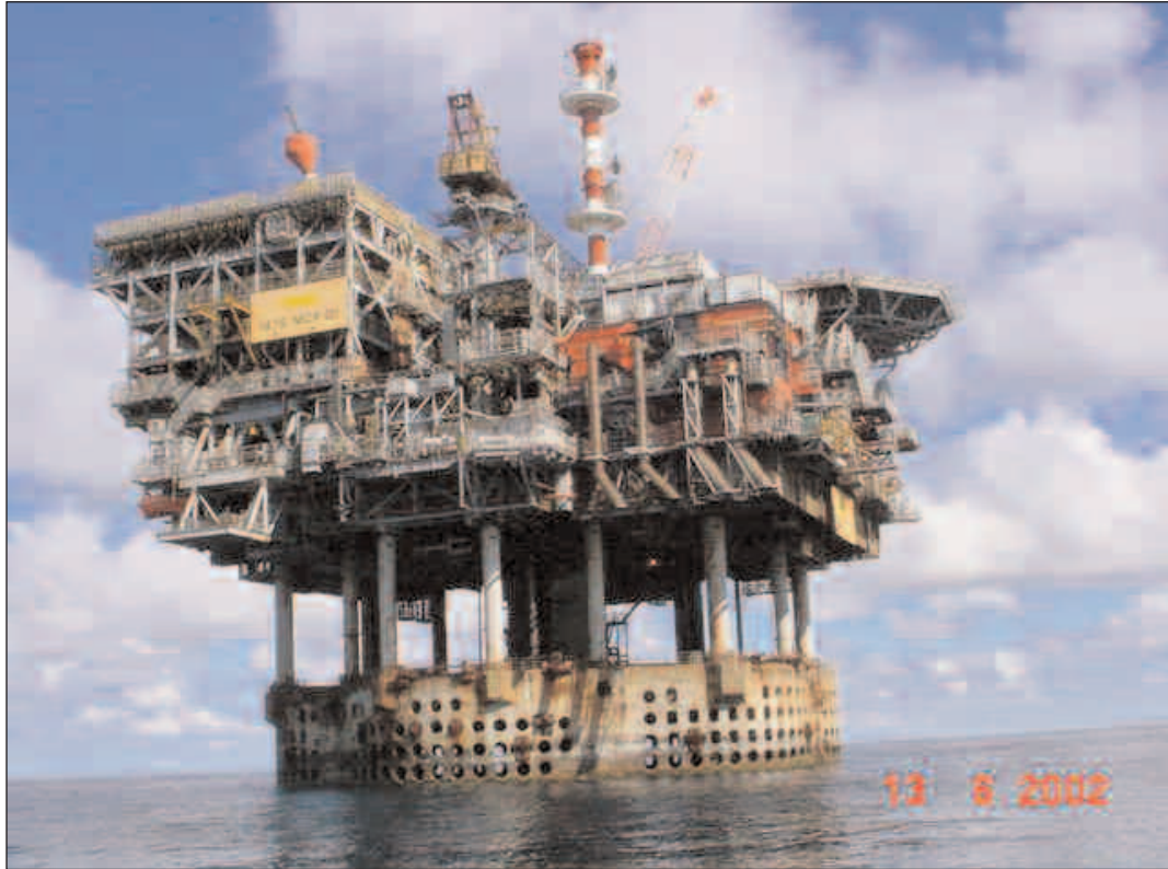
Figure 3.1 Manifold and Compression Platform MCP-01
