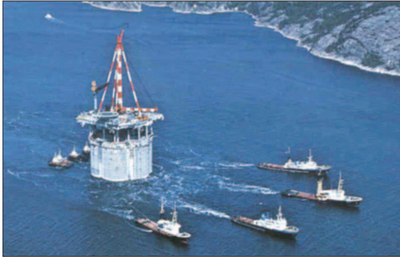
Figure 6.3 Tow-out of MCP-01 in 1976
