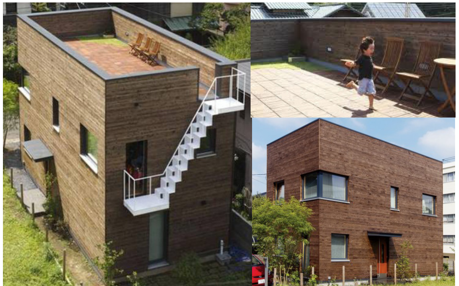
Fig. 16, 17, 18 Kamakura House - Exterior views.
